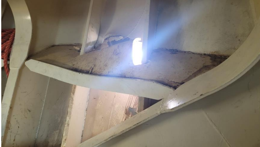
Image 5 - Damage observed from the interior frame of the Tradewind Passion
